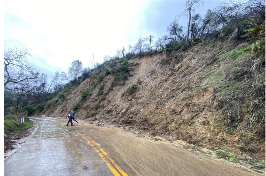
Pleasants Valley Road during severe storms in Unincorporated County
