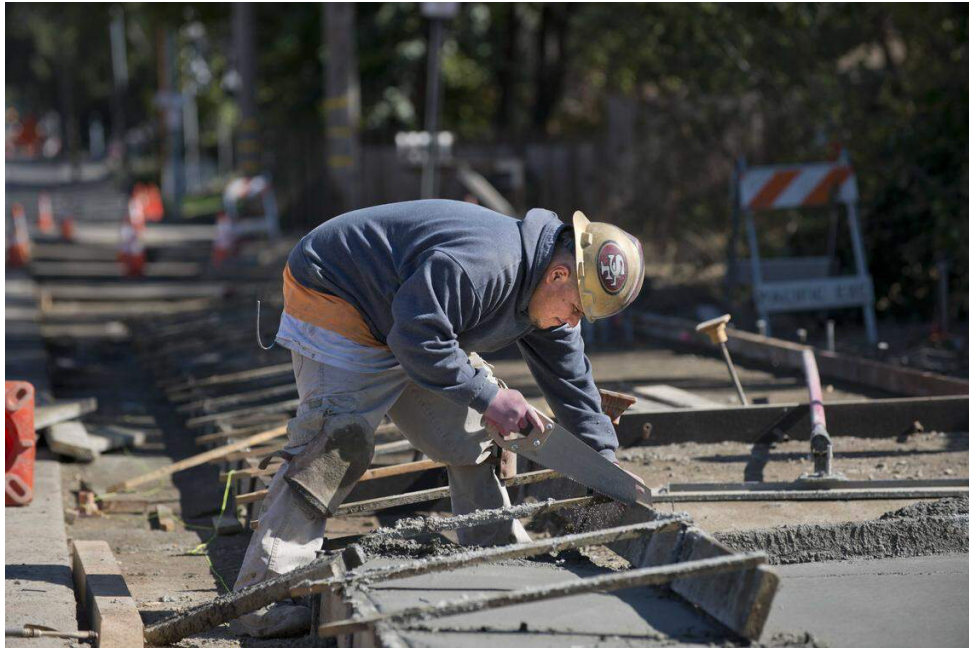
A construction worker cuts lumber while building a sidewalk along Marconi Avenue in Carmichael in 2013. Sidewalk construction projects like this are often built in phases as local agencies compete for limited state Active Transportation Program grants to fund pedestrian safety improvements. Hector Amezcua hamezcua@sacbee.com
