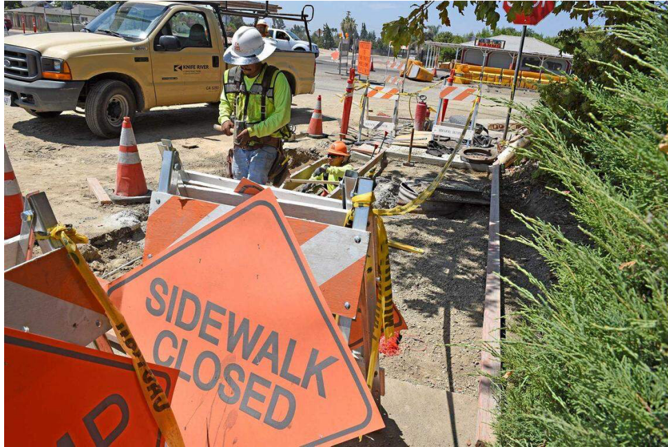
A construction worker builds a sidewalk on Chicago Avenue at Carpenter Road in Modesto in 2018. Dozens of pedestrian safety projects across California have remained unfunded after the state reduced support for the Active Transportation Program in 2024. Joan Barnett Lee Modesto Bee file
