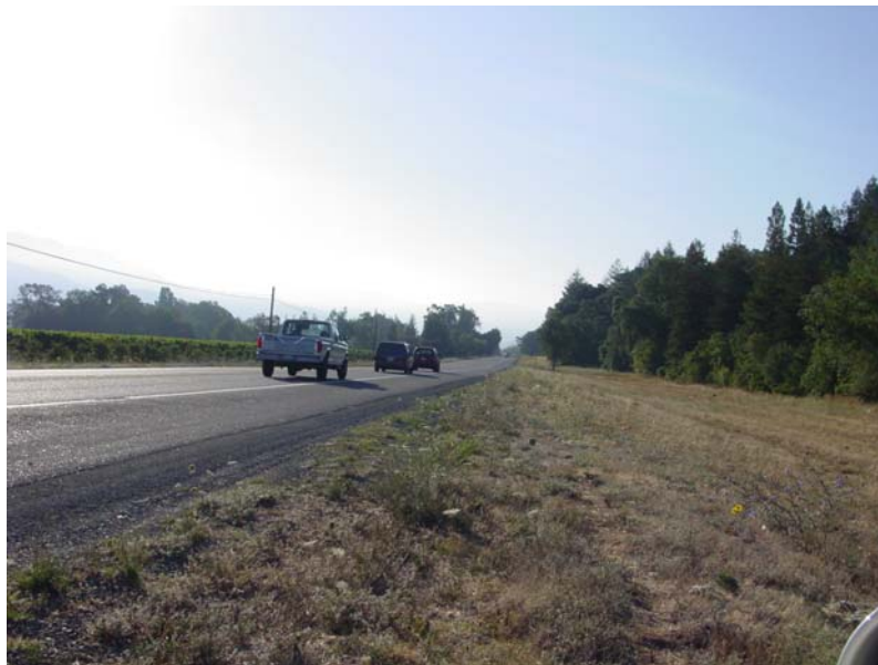
SR 29 ROW—Note that space is available on the side.
