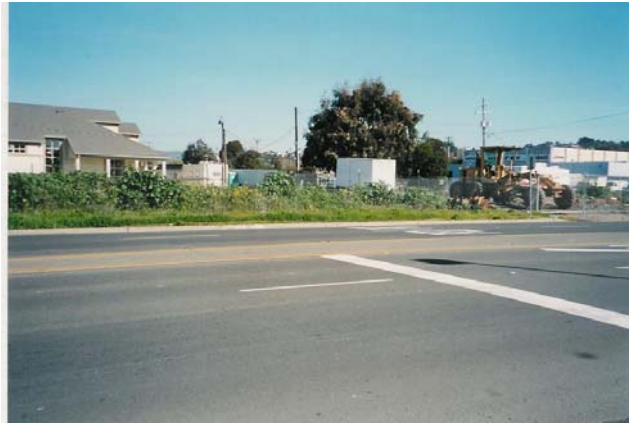
Photo 10-Nine Sereno Transit Center Site
