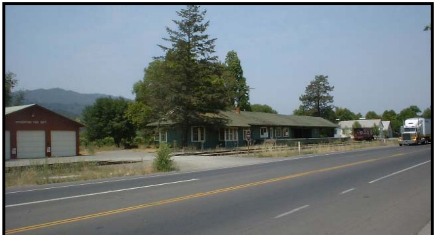
View of the historic depot building on the potential Rutherford station site from the intersection of Highway 29 and Rutherford Cross Road.
