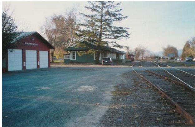
Photo 10-Twenty-One Rutherford Station Site
