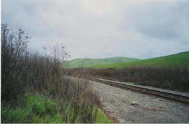
Photo 10-Five Creston Siding – Solano County
