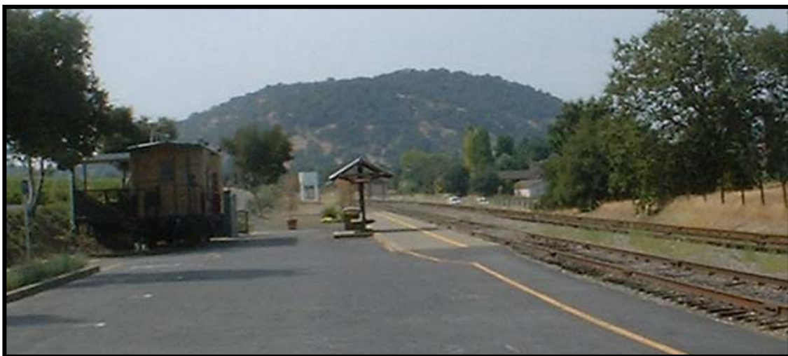
Existing Yountville Wine Train Station at California Avenue.
