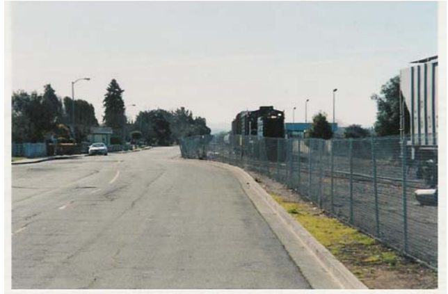
Photo 10-Ten Tracks South of Tuolumne Street
