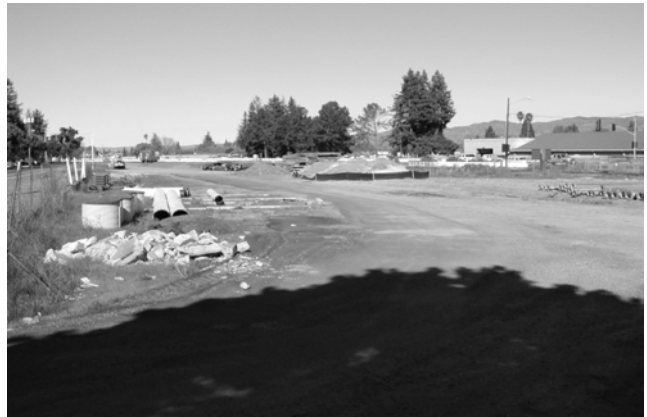
Photo 10-Eighteen North Napa Station Site Looking North
