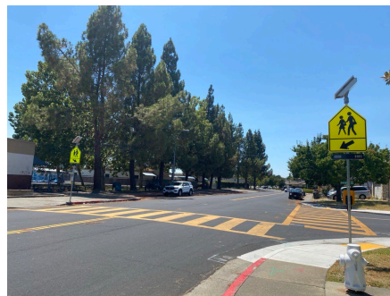
Completed RRFB installation at Cement Hill Road
