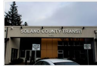
SolTrans Operations & Maintenance Facility
