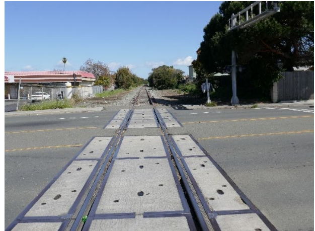
Figure 11 - CFNR-Sereno Grade Crossing
