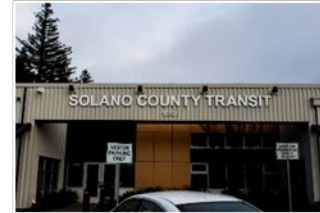
SolTrans Operations & Maintenance Facility
