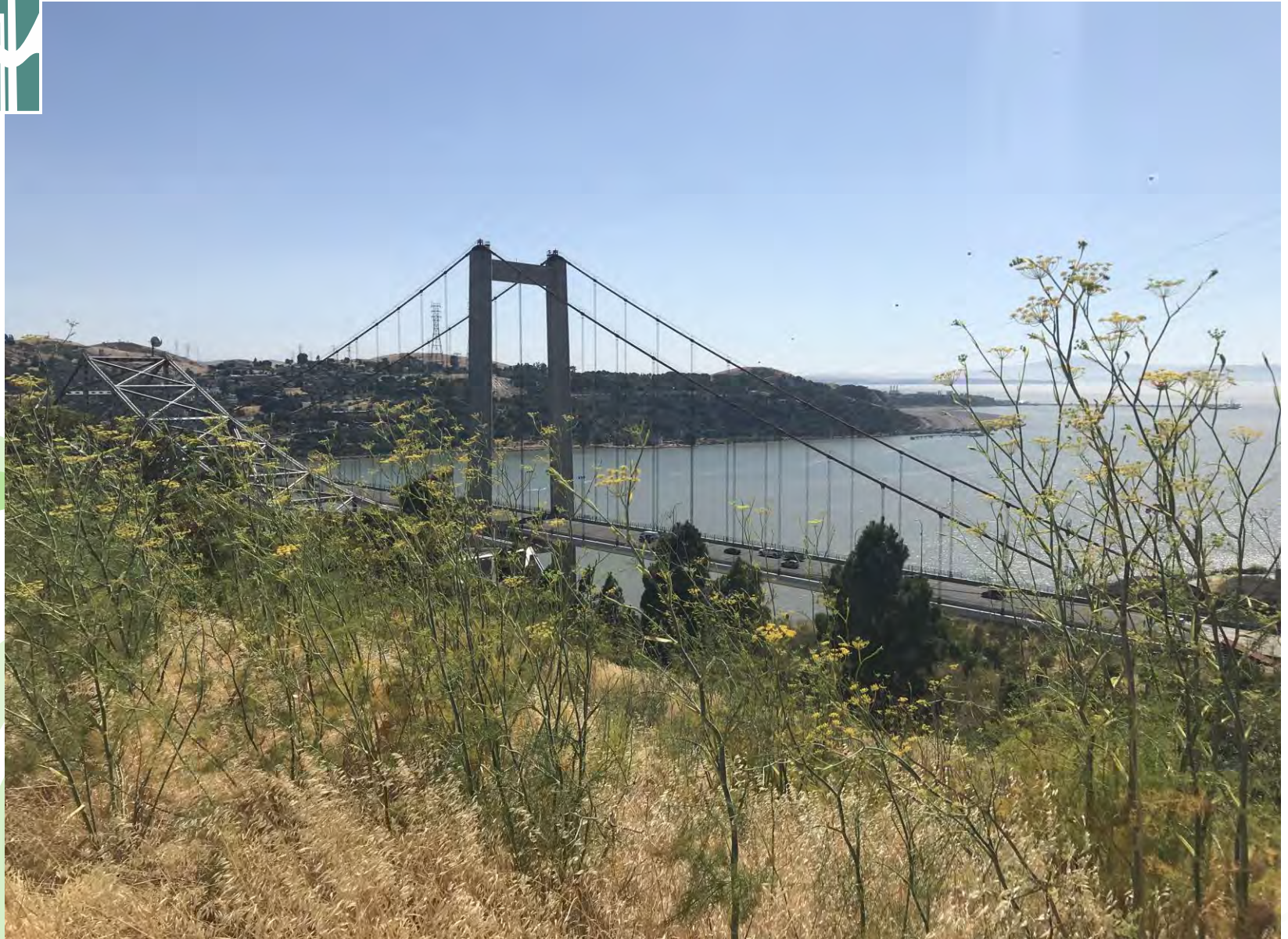
View of the Carquinez Bridge from the top of the Vallejo Bluff (looking southwest)
