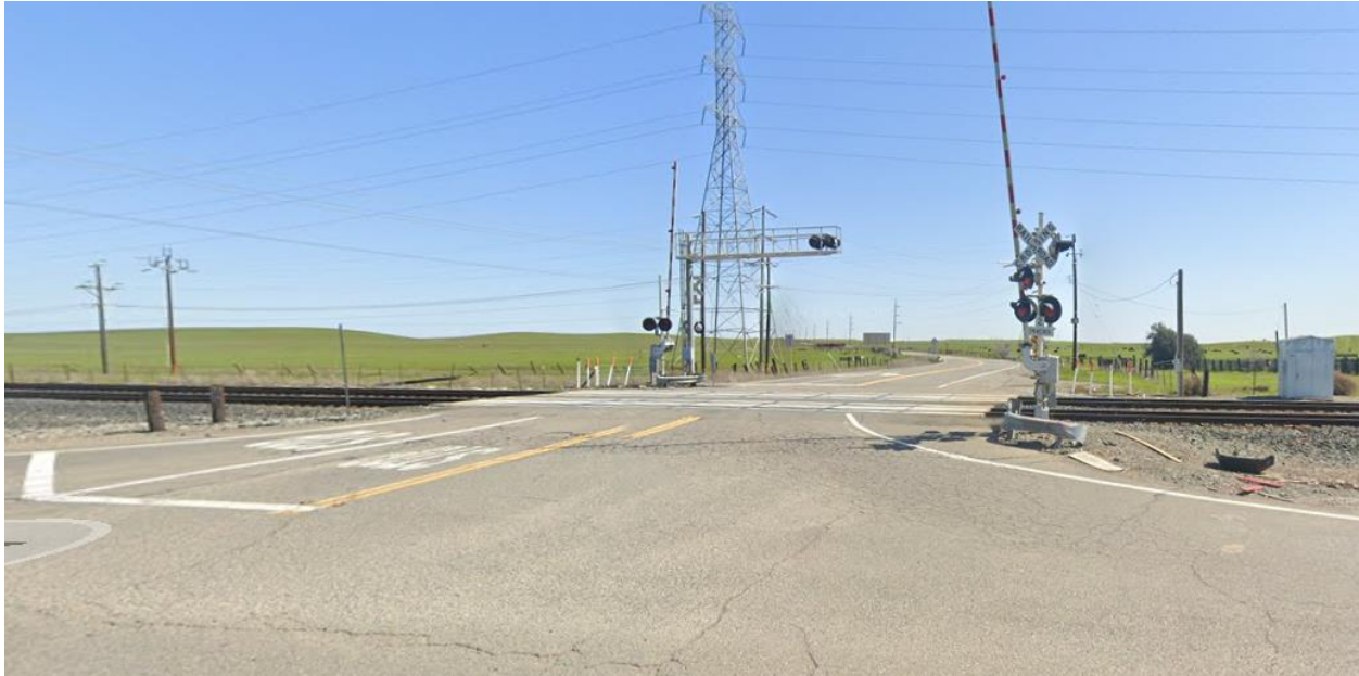
Canon Road Looking West
