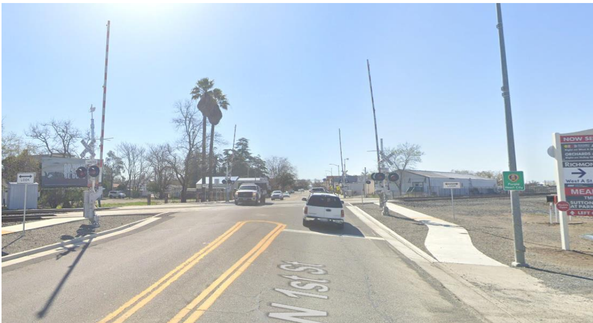
1 st Street Looking South
