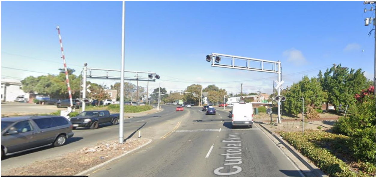
Curtola Pkwy Looking West
