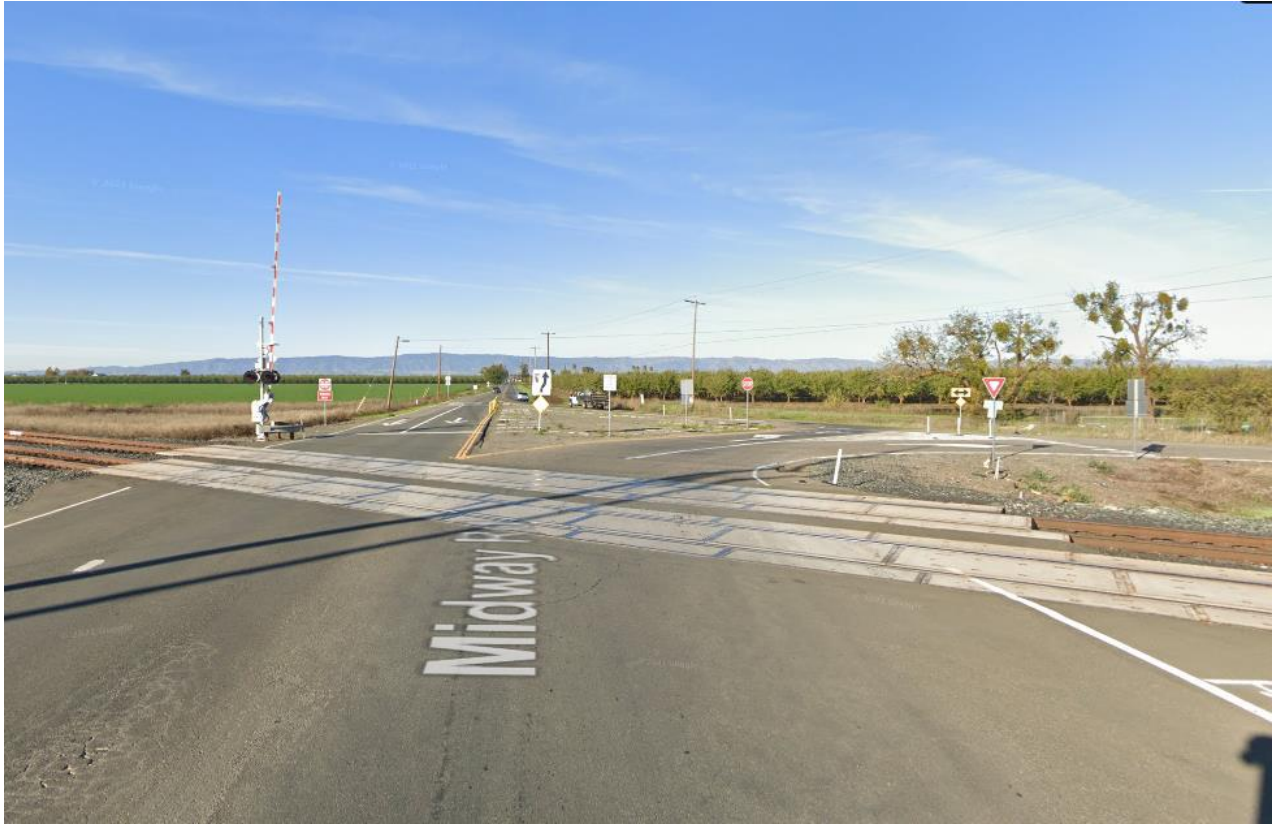
Midway Road Looking West
