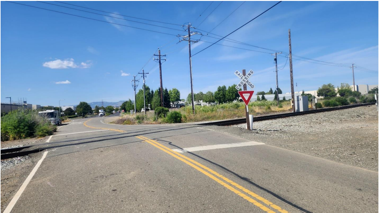
Chadbourne Rd Crossing
