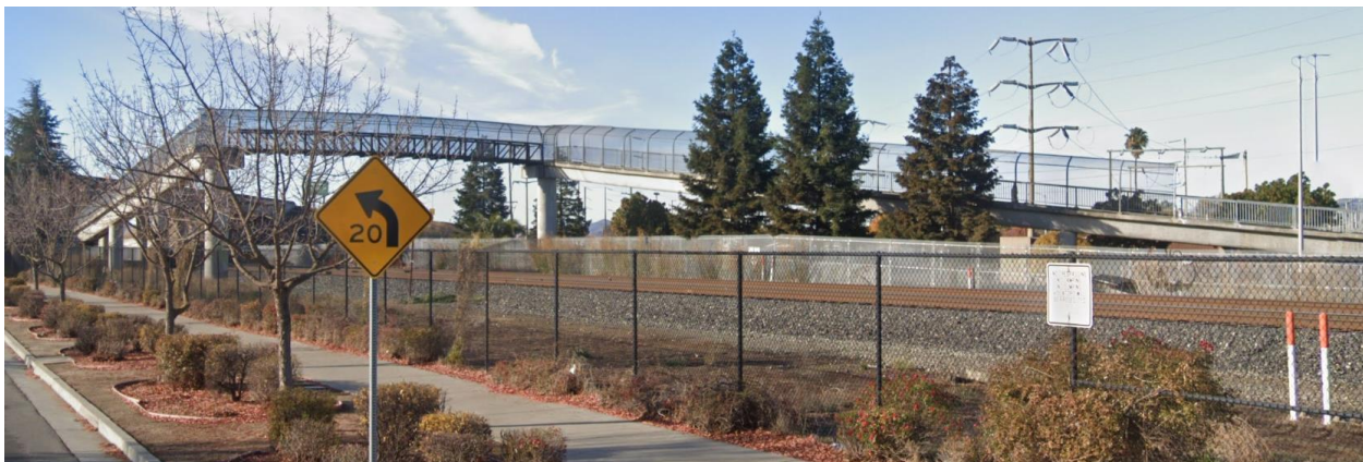
Suisun-Fairfield Amtrak Station Existing Bike and Pedestrian Bridge (from Suisun City, northeast of Station)
