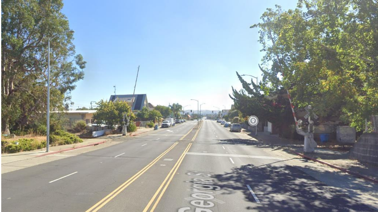
Georgia Street Looking East
