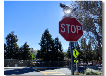
Installed RRFB. Funding awarded to Joe Henderson Elementary School (Benicia) from Cycle 1.
