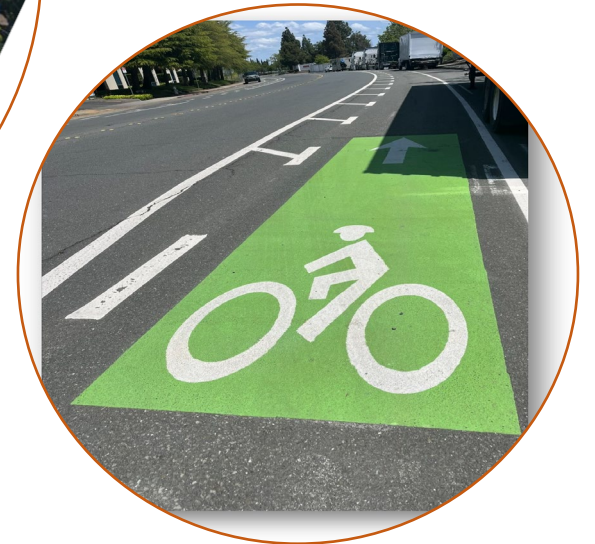
Suisun City- Rail Road Avenue Pavement Rehabilitation Project
