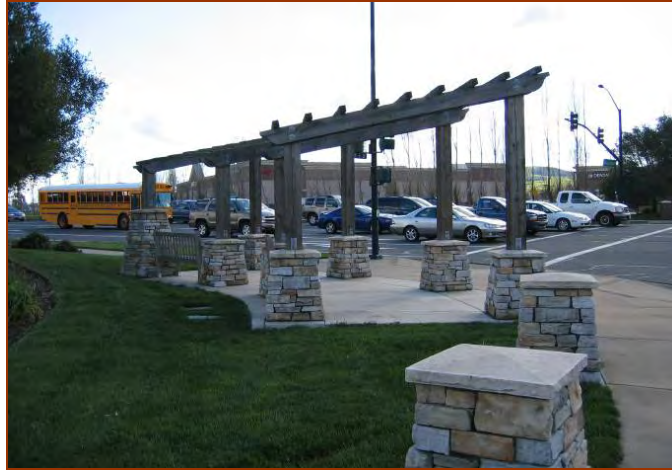
Photo: Elements of a rest stop on Business Center Drive
