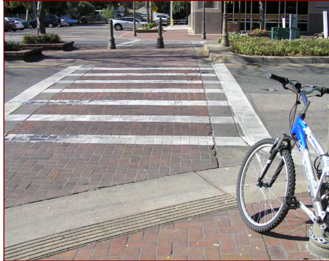
Photo: "Ladder" crossing (also with different pavement material)
