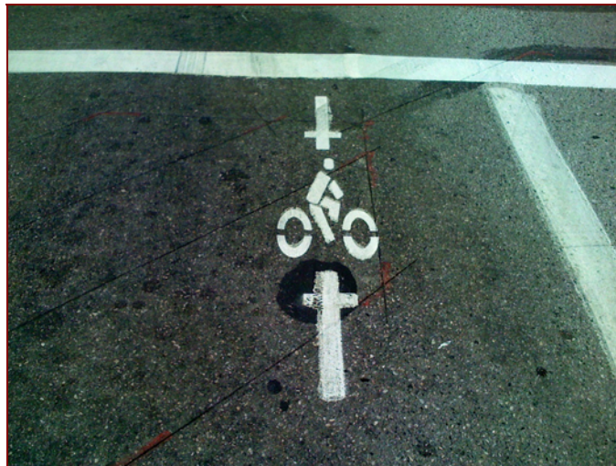
Photo: Bicycle detector at an intersection
