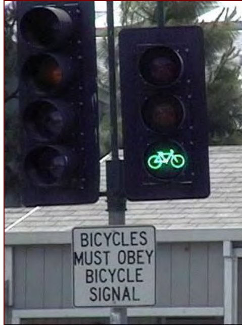
Photo: Signal designated for bicycles
