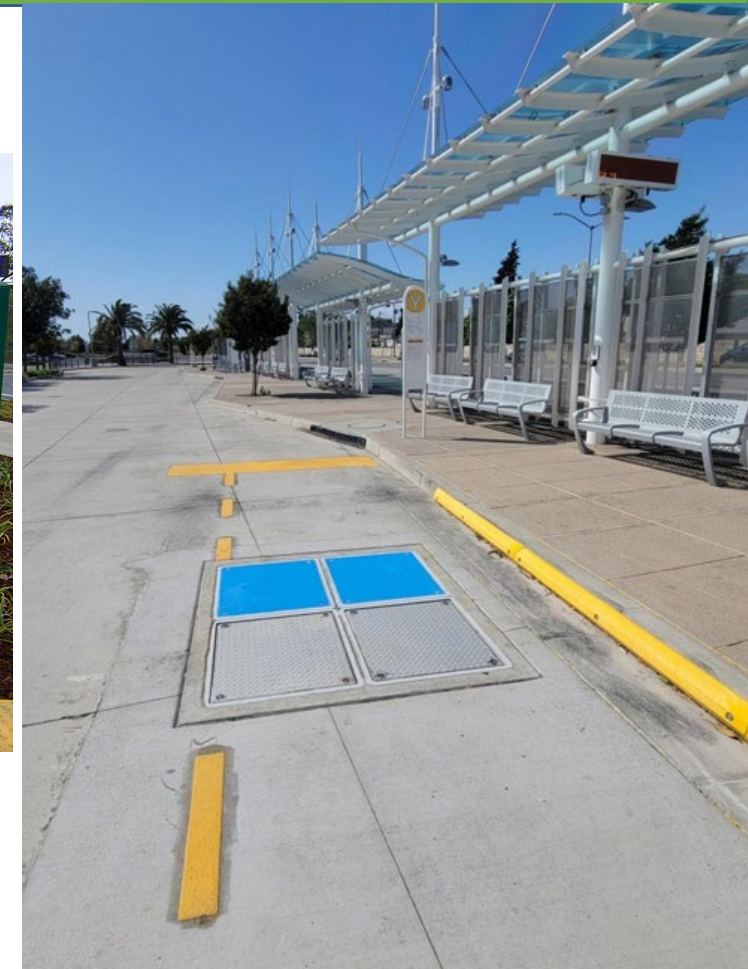
Curtola Park & Ride Lot Expansion and Inductive Charging
