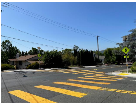
Rapid Flashing Beacons at East 2 nd Street and Riverhill Drive, Benicia
