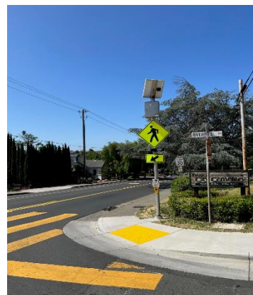
Rapid Flashing Beacons at East 2 nd Street and Riverhill Drive, Benicia
