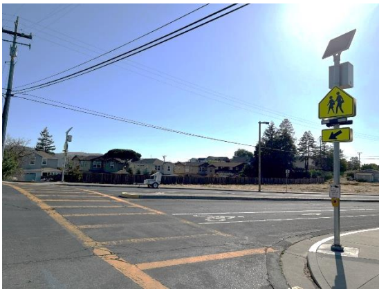
Rapid Flashing Beacon – Denfield Way and Military West, Benicia
