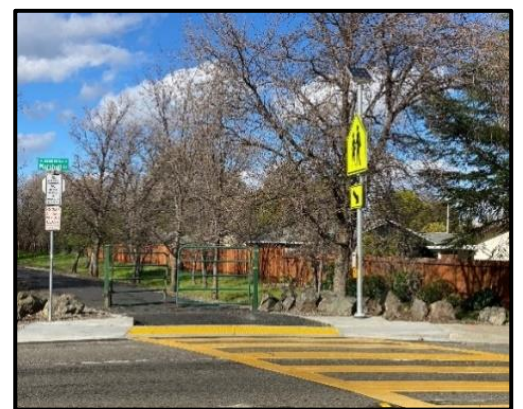
HSIP 9 crossing improvements at the Southside Bikeway crossing and Marshall Road (Vacaville)
