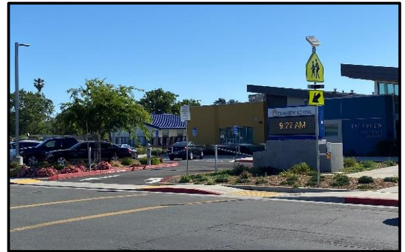
Rectangular Rapid Flashing Beacons were installed at Fairview Elementary (Fairfield). This location was identified for an improved crossing with a SR2S walk audit and discussion within the Fairfield 3Es Committee.
