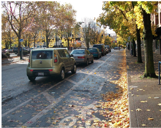
Figure 1. Poorly maintained buffered bike lane covered in leaves that could cause a bicyclist to slip and fall.
