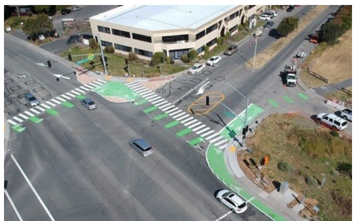
Figure 1. Rapid installation bicycle and pedestrian crossings at the intersection of Central Avenue and Rydin Road in Richmond, CA
