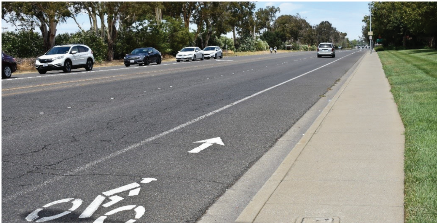
Figure VC-3: Bike Lane in Vacaville
