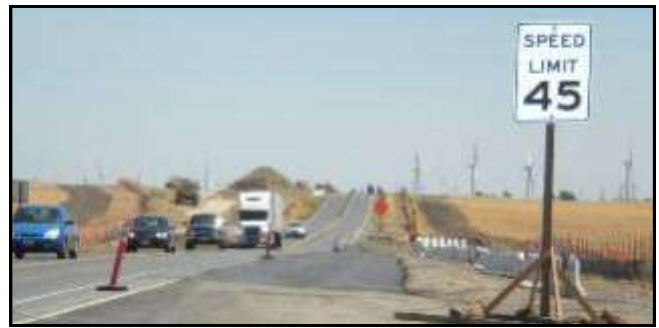
Lane Widening Construction on SR 12 East
