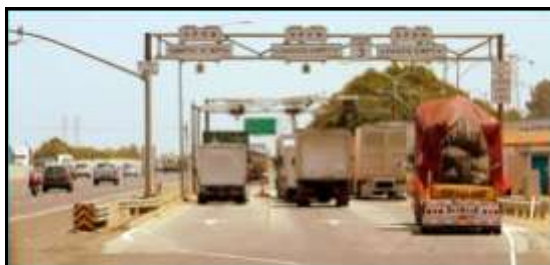
I-80 Eastbound Truck Scales (Existing)
