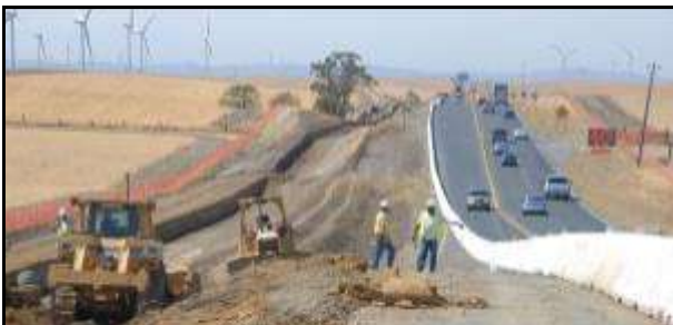
Lane Widening Construction on SR 12 East
