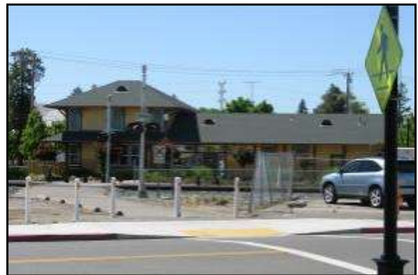
Current West B Street At-Grade Rail Crossing
