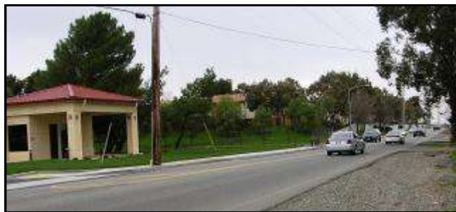
Travis AFB North Gate Access
