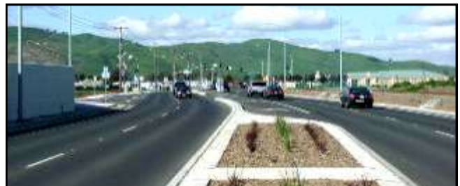
Jepson Parkway—Walters Road Widening, Suisun City
