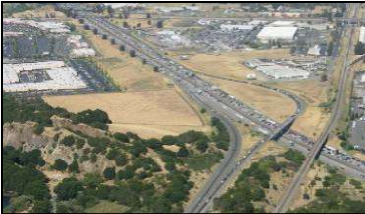
I-80/I-680/SR 12 Interchange Complex
