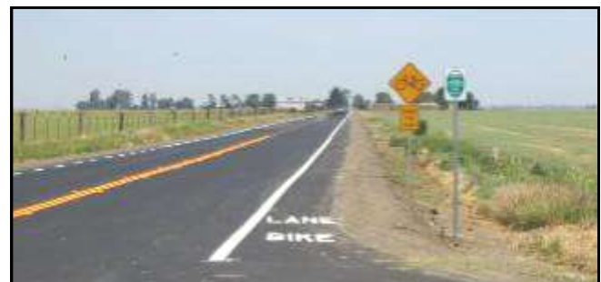
Completed Vacaville-Dixon Bicycle Route, Phase 3
