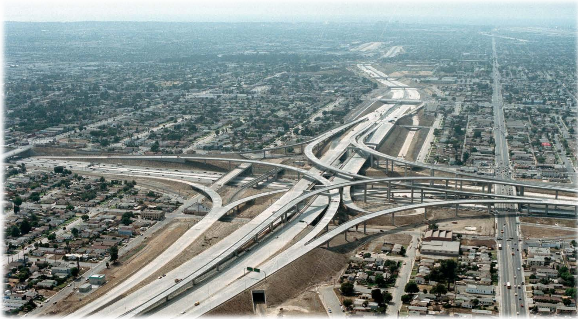
I-105/405 interchange bisecting four communities in Los Angeles, CA. Source: California Department of Transportation
