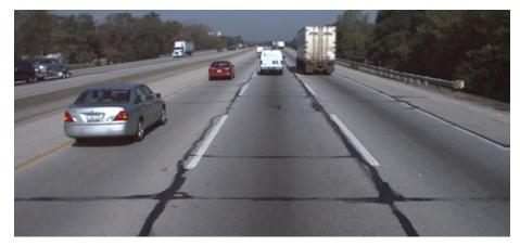
Concrete slab faulting is determined by Caltrans engineers who measure the faulting height and number of faults. To monitor the pavement smoothness, a Caltrans vehicle gathers accurate data from speeds of 10 miles per hour (mph) up to 70 mph and the IRI is
