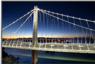
San Francisco-Oakland Bay Bridge Opened 1936 New East Span Opened September 2013
