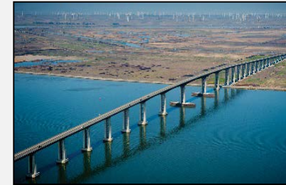
Antioch Bridge Opened 1926 Replaced 1978
