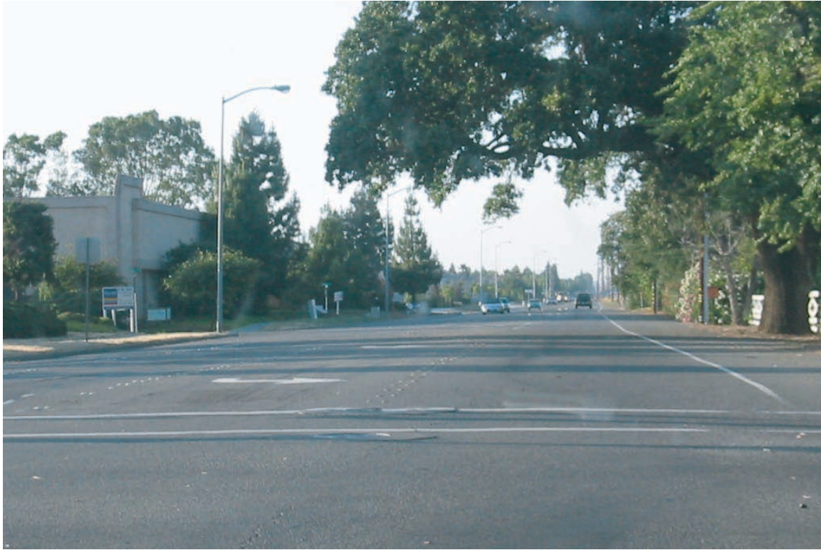
a. North-facing view on Leisure Town Road at Elmira Road.
