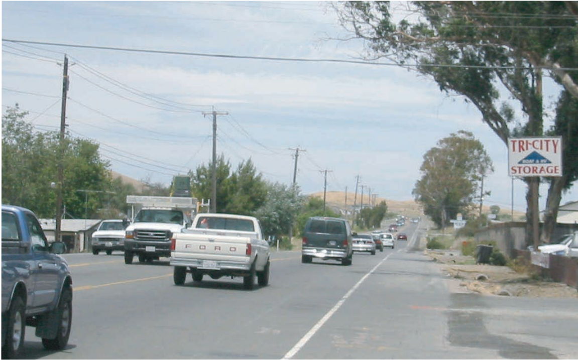
a. North-facing view on Peabody Road north of Cement Hill Road.
